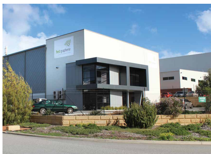
100 tonne/year manufacturing facility at Henderson, WA
