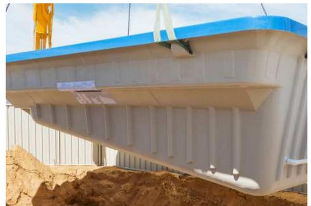
Fig.2 – Monoblock fibreglass in-ground swimming pool
