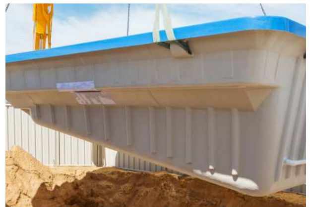
Fig.2 – Monoblock fibreglass in-ground swimming pool
