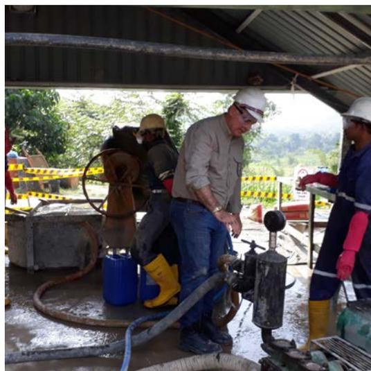
Figure 1: Managing Director, Craig McGuckin, providing instruction on pressure grouting at Shaft H
