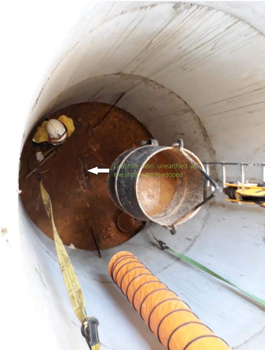
Figure 3: Shaft J 2.5 metres liner showing weathered graphite vein in shaft
